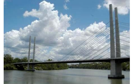
Lady Eleanor Schonell Bridge, Brisbane 1 x Zincode 402 @ 75 microns 2 x Ferreko No 3 @ 100 microns per coat
