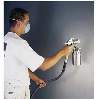
Spray application of waterborne metallic paint. Polyurethane paint requires full air-fed head gear.
