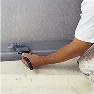
Application by roller or brush generally results in a **vastly different finish** from that of spray application, as the metallic pigment particles are highly irregular in shape, and therefore **inhibit the natural flow-out** of the wet paint. The movement of the brush or roller also alters the orientation of the flake pigment. For this reason, metallic paints exhibit higher brush-marking, roller-marking and stipple than other types of paint.
