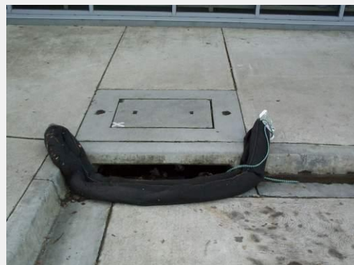
Peat Sorb positioned to block the spill. Quick action is required to position the plug to contain the spill
