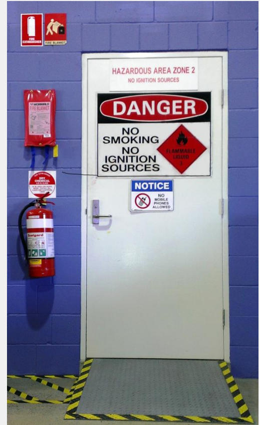
A typical bund room door in a Dulux Trade Centre. Note the warning signs and fire equipment.
