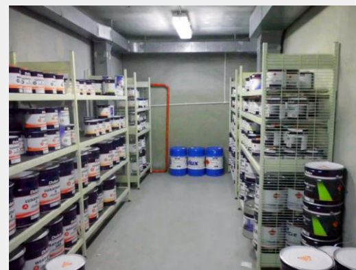
A good bund room also features ventilation and sturdy racking, and is neat and free of clutter.
