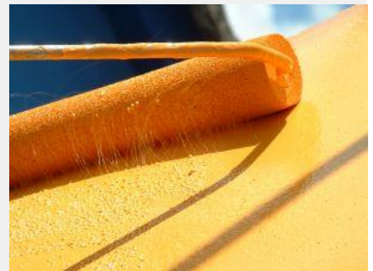
Without a solvent that extends drying time, paint dries too quickly during application, and becomes too thick and stringy to allow a good finish.
