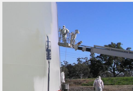
Even if spraying out in the open in extremely well ventilated environments, it still makes sense to protect yourself!
