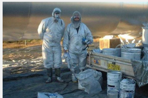
These applicators safely coated the Warragamba pipeline with Dulux Protective Coatings
