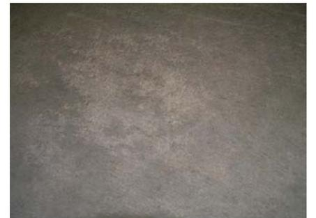
Laitance & roughness on concrete
