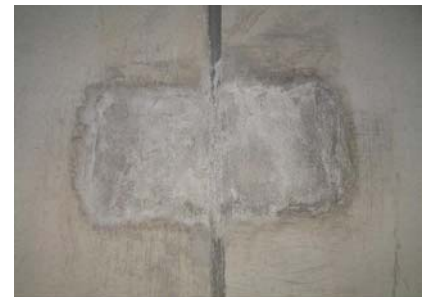
Repair patch showing laitance
