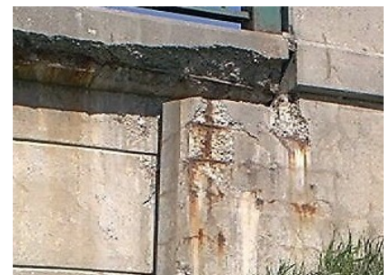
Repair patch showing laitance
