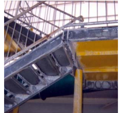
Severe zinc depletion of HDG steel in a new swimming centre. Red rusted areas indicate complete zinc layer depletion and steel corrosion. Extensive rectification work delayed the opening of the pool and blew out project costs.
