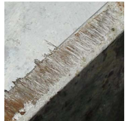
Severe zinc depletion of HDG steel in a new swimming centre. Red rusted areas indicate complete zinc layer depletion and steel corrosion. Extensive rectification work delayed the opening of the pool and blew out project costs.
